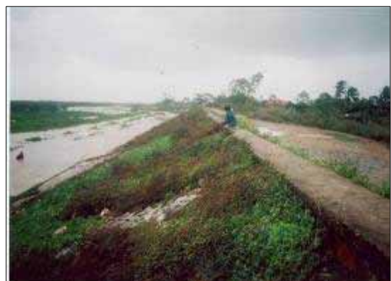
Fig. 11. Soil sea dykes protected by mangrove stretches remained intact
