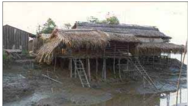
Fig. 2. Roof thatching by nipa palm shingles
